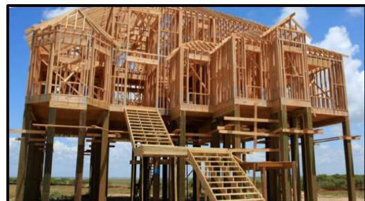
Figure 123 Elevated Substructure for flood prone areas
