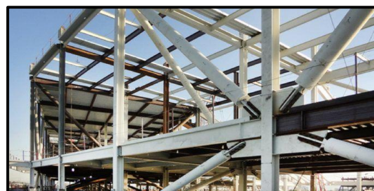
Figure 124 Diagonal Bracing against Wind loads
