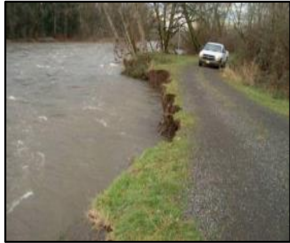
Figure 23 Example of soil erosion due to flow of water
