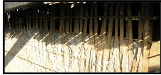
Figure 110 Wattle and Daub Method
