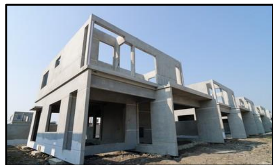
Figure 115 Grey Structure of Pre-cast concrete
