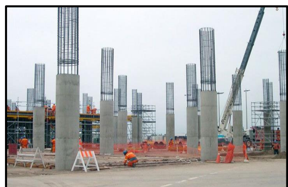
Figure 117 RCC Columns of Building
