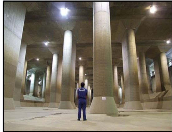
Figure 62 Underground Discharge Channel Tokyo, Japan
