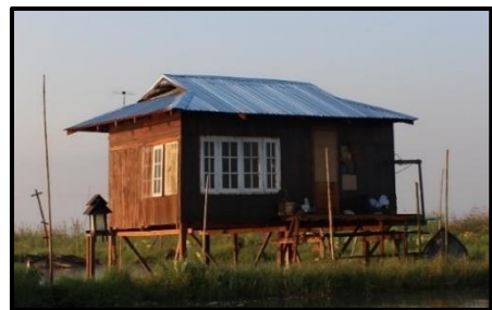
Figure 46 Example of elevated house
