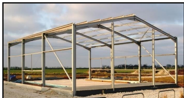
Figure 54 Galvanized Steel Structure
