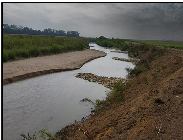
Figure 102 Channel Modification to regulate flow of water
