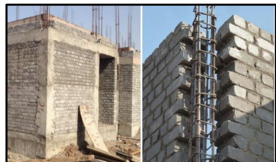
Figure 116 Steel Reinforcement in confined masonry structures
