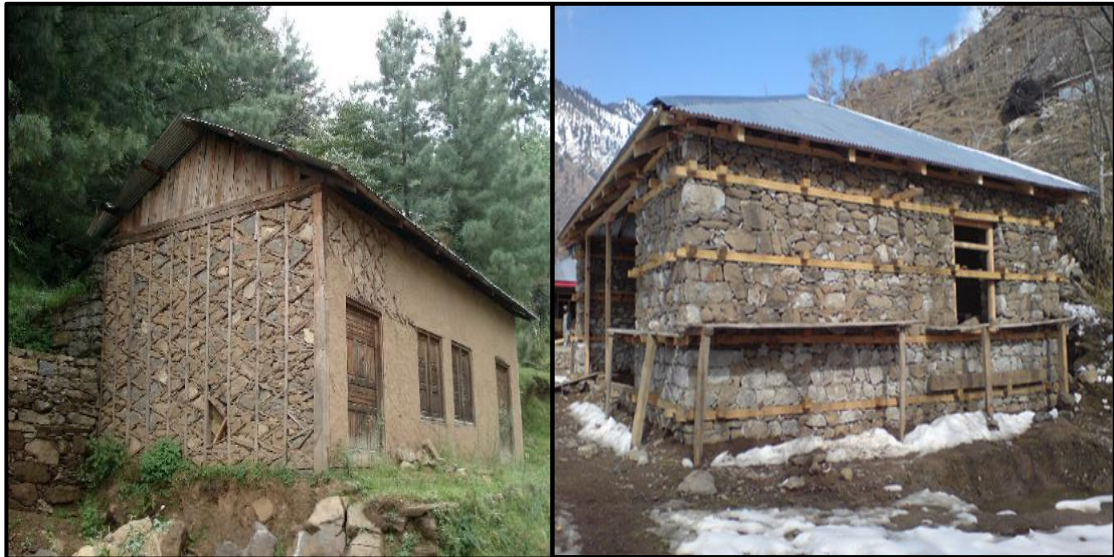
Figure 94 Improved Stone Masonry Construction for Mountainous Areas
