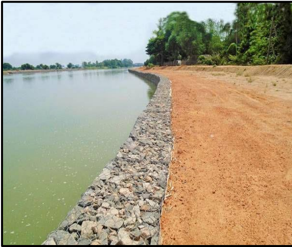
Figure 22 Riverbank Protection Works for Vennar River
