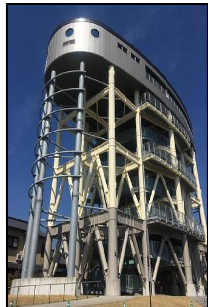
Figure 61 SAGA AREA Tsunami Evacuation Tower
