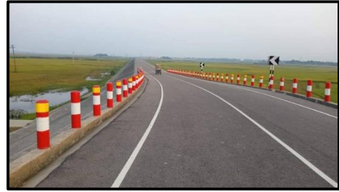
Figure 49 Example of Raised Roads
