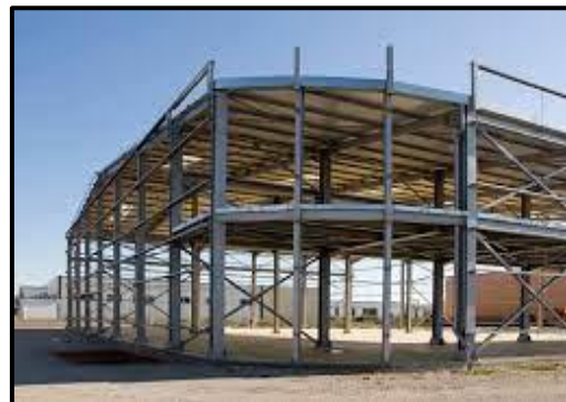
Figure 121 Galvanized Steel Structure
