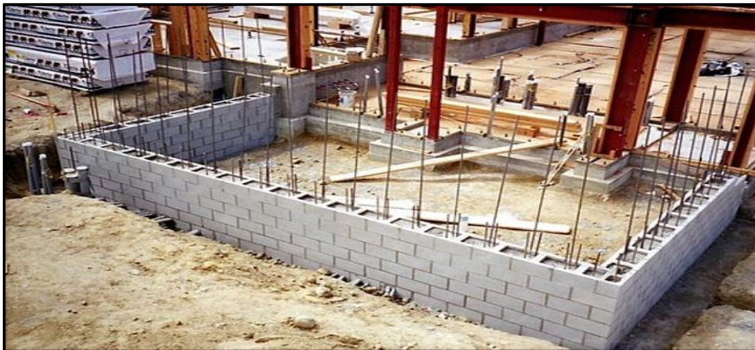
Figure 93 Steel Reinforcement in Confined Concrete Block Masonry
