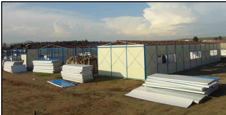
Figure 92 Sample of Prefabricated Structure
