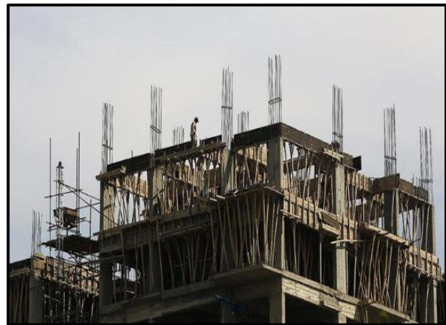
Figure 98 Steel Reinforcement for RCC Construction of High-Rise Structure
