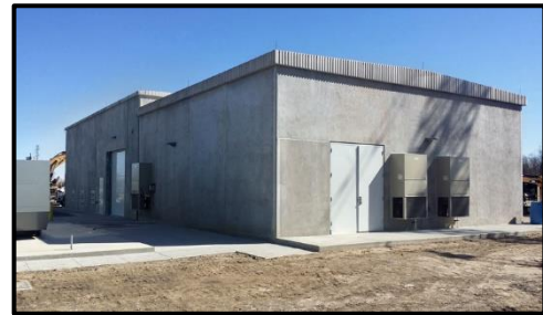
Figure 125 Precast Concrete Structure
