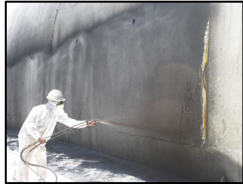
Figure 122 Bitumen coating for water proofing of structures
