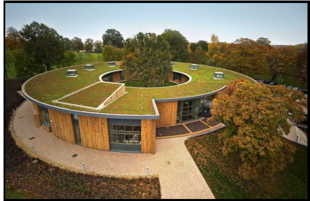
Figure 107 Example of Green Roofs on building.
