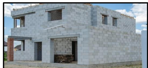
Figure 128 Concrete Block Masonry
