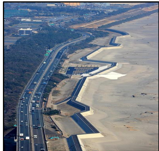
Figure 59 Shizuoka Prefecture-A massive Seawall to prevent flooding
