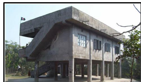
Figure 47 Elevated shelter at Rayenda union of Bagerhat district
