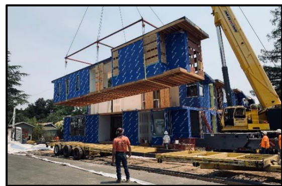
Figure 14 Example of Modular Construction
