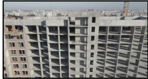
Figure 127 RCC High Rise Grey Structure
