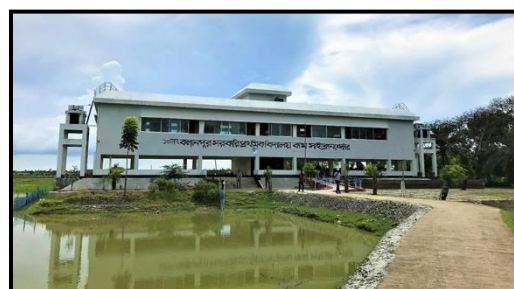
Figure 67 Multipurpose Disaster Shelter in Shatkhira, Bangladesh
