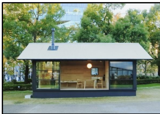
Figure 15 Example of modular construction, MUJI Hut, Japan
