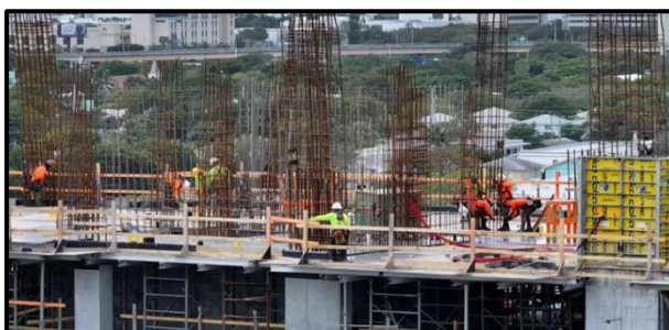
Figure 99 Steel Reinforcement for RCC Structures High Rise Buildings
