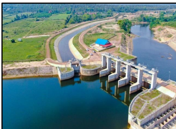
Figure 42 Water management through Barrage
