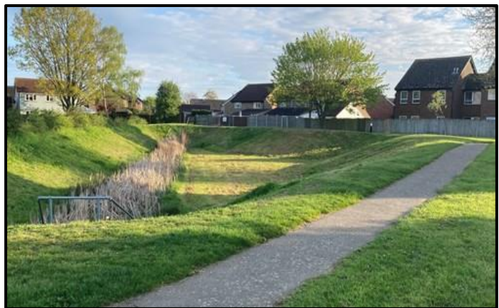
Figure 106 Detention Basins to tackle flood mitigation
