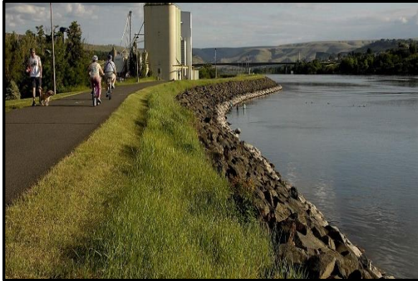
Figure 37 Levee Built as an embankment along the river course
