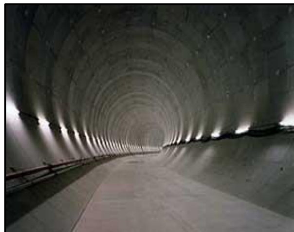
Figure 63 Underground connecting tunnel for flow channel, Tokyo Japan
