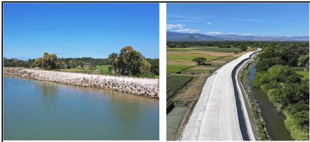
Figure 44 Example of sea dike and embankment
