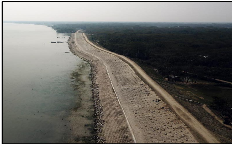
Figure 64 Coastal Embankment Improvement (Phase-01) of Project
