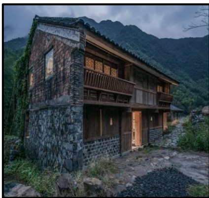
Figure 17 Example of Wooden Reinforced Stone Construction in China
