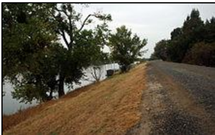
Figure 24 The side of a levee in Sacramento, California
