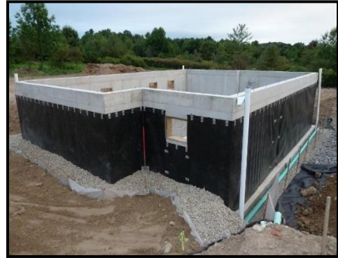
Figure 55 Water proofing treatment
