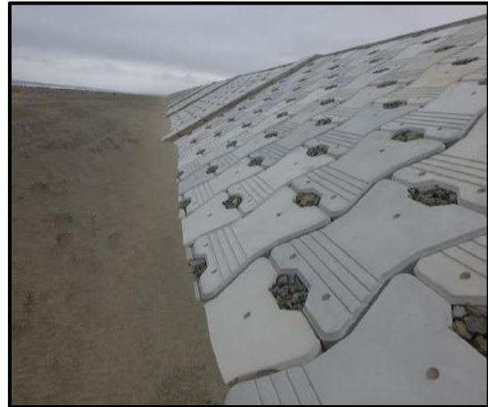
Figure 60 Sendau Airport Japan Sea Dike
