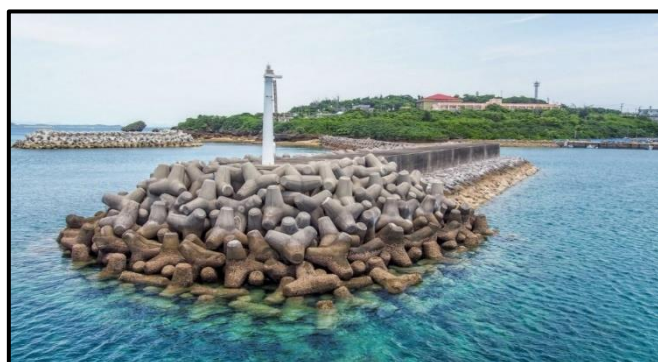
Figure 58 Tsukenjima Breakwater Lighthouse, Japan
