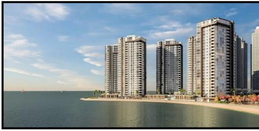
Figure 51 High Rise Construction
