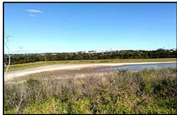
Figure 38 A detention basin in Western Sydney, Australia
