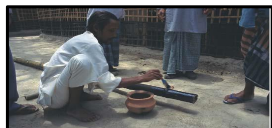
Figure 109 Bitumen coating on structural element
