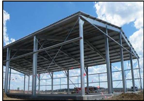
Figure 97 Sample of Pre-Engineered Buildings
